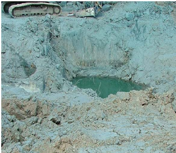
Stabilized foundation and soils with uranium and fission product contamination.
