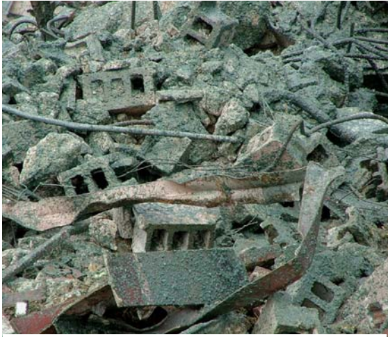
Stabilized demolition debris with uranium and fission product contamination.
